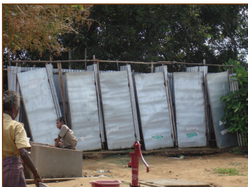
Toilets in the temporary shelter complex
